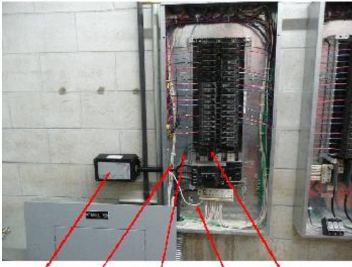
SPD Ground Phases Neutral Breaker
